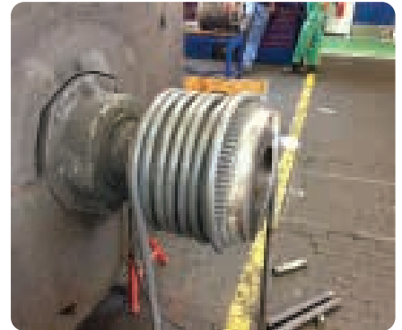
Heating a coupling for dismounting
